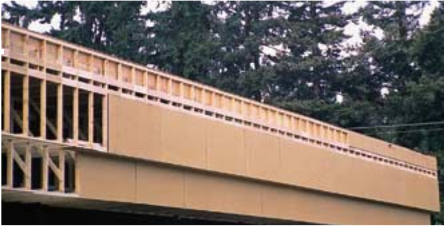
MDO panels create a smooth, easy-to-finish surface in fascias.
