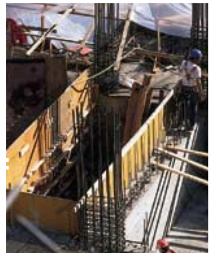
HDO panels can be reused many times in concrete forming.
